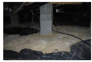
Engineered Lumber. FRAMING: OSB. **SUBFLOOR** BEAMS: TYPE Wood. **BEAMS - CONDITION:** Appear functional. Appear functional. FLOOR JOISTS: COLUMNS/SUPPORTS: TYPE Cinderblock. Appear functional.
